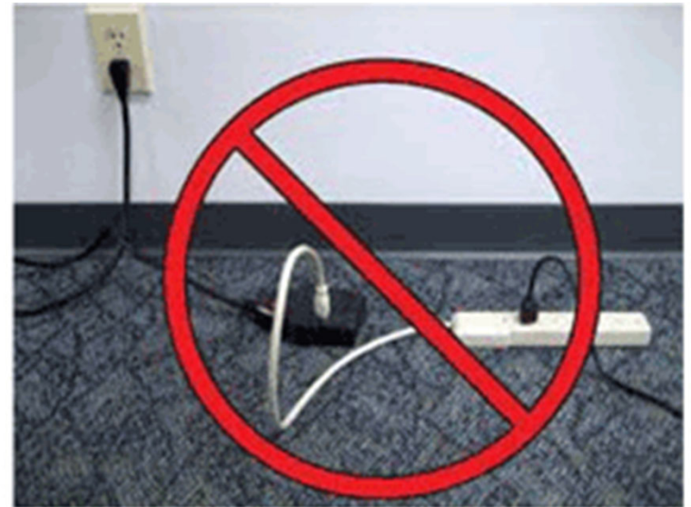
Daisy-chained multi-plug outlets
